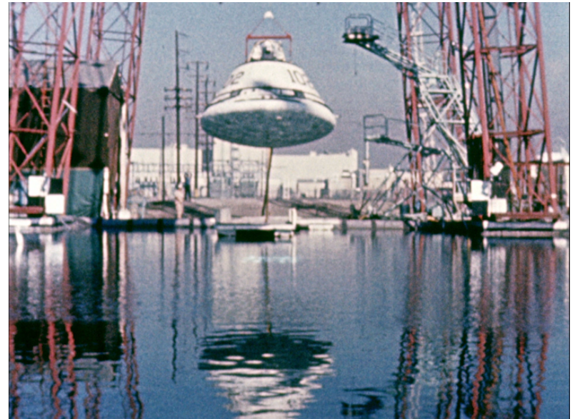
Full-scale splashdown tests at North American Aviation
